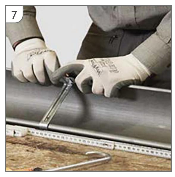
Clip concealed brackets to the cut lengths of gutter at 400mm max centres.
