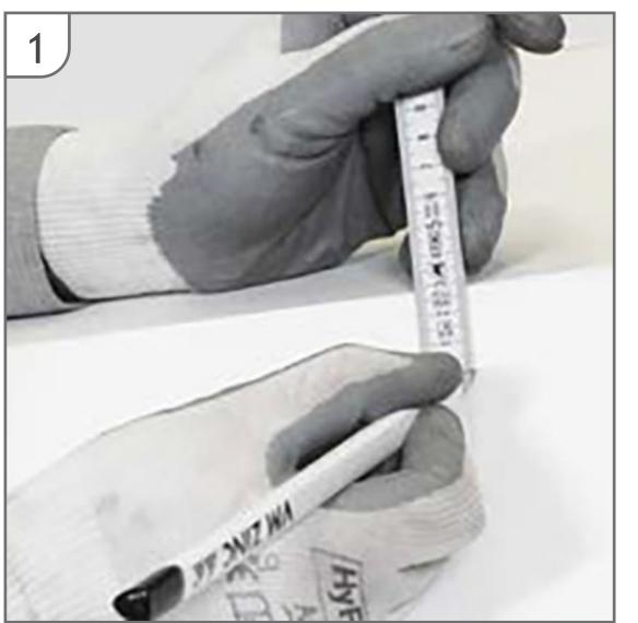
Using a rule, make a chalkline setting the fall (min 1:200) towards the running outlet and required position of the downpipe.
