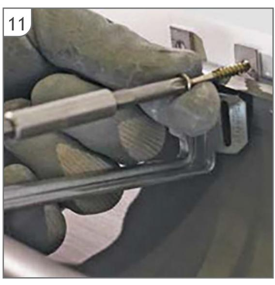
Fix the gutter brackets according to the chalkline.
